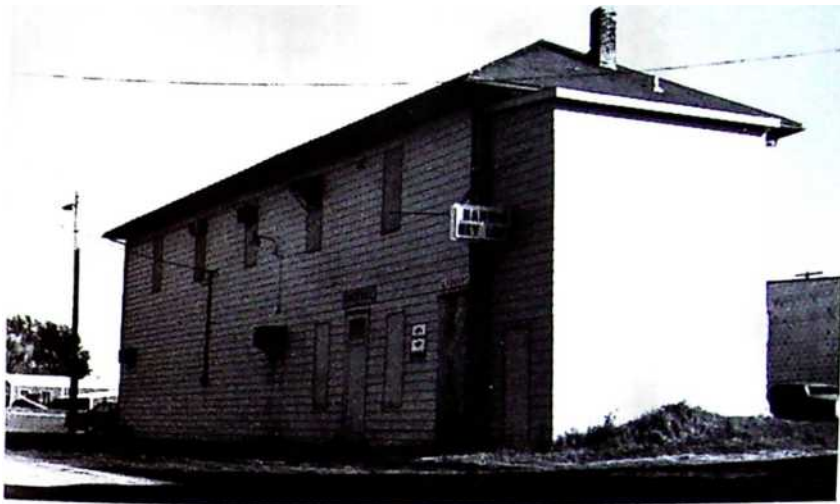
This was the old Victor Johnson building. Notice the “Harris Hey o sign. That is the door that was the entrance to the Jarchow Hall which or many years was the entertainment center and place for meetings.
