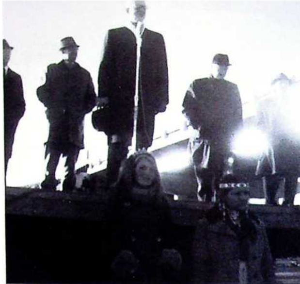
Governor Harold LeVander speaking at the opening of Interstate 35 at the Harris intersection on November 25, 1969.
