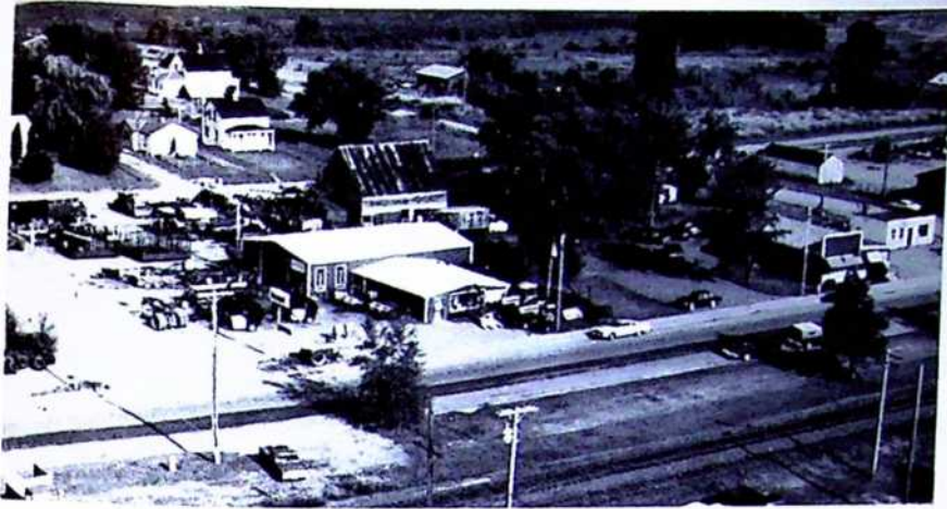
Looking southeast, a view of Wayside Equipment with the old livery barn in the background.
