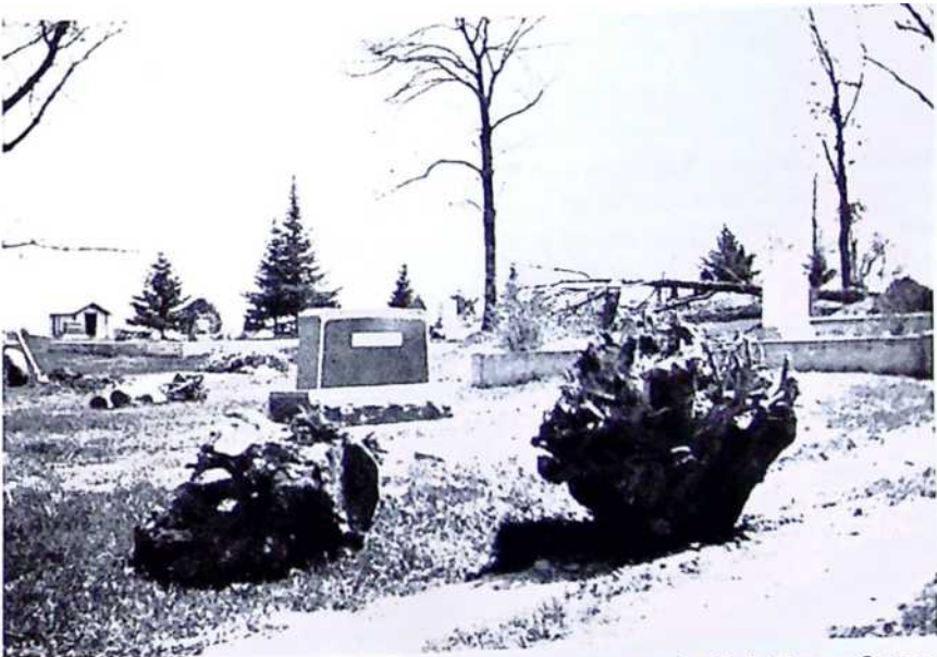
A 1936 W.P.A. project; digging out oak stumps at the Oak Grove Ceme-
